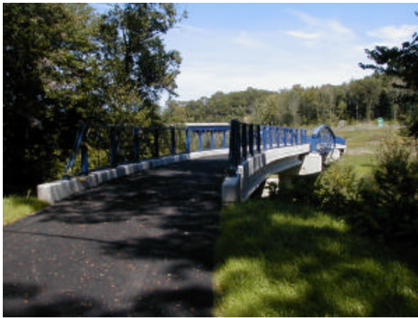
Completed section within the Rt 146 project...
