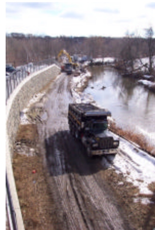
Bikeway construction in Worcester near Rt. 20.
