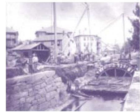
**When the Blackstone Canal Company folded, parts of the abandoned trench deteriorated into rank open sewers. During the 1890s, they were sensibly integrated into Worcester’s underground waste water system. Dressed granite blocks from the 13-foot walls of the 82-foot long locks were sold and carted away to become parts of new buildings. During deep excavations, the city’s highway department even now sometimes uncovers the canal.**
